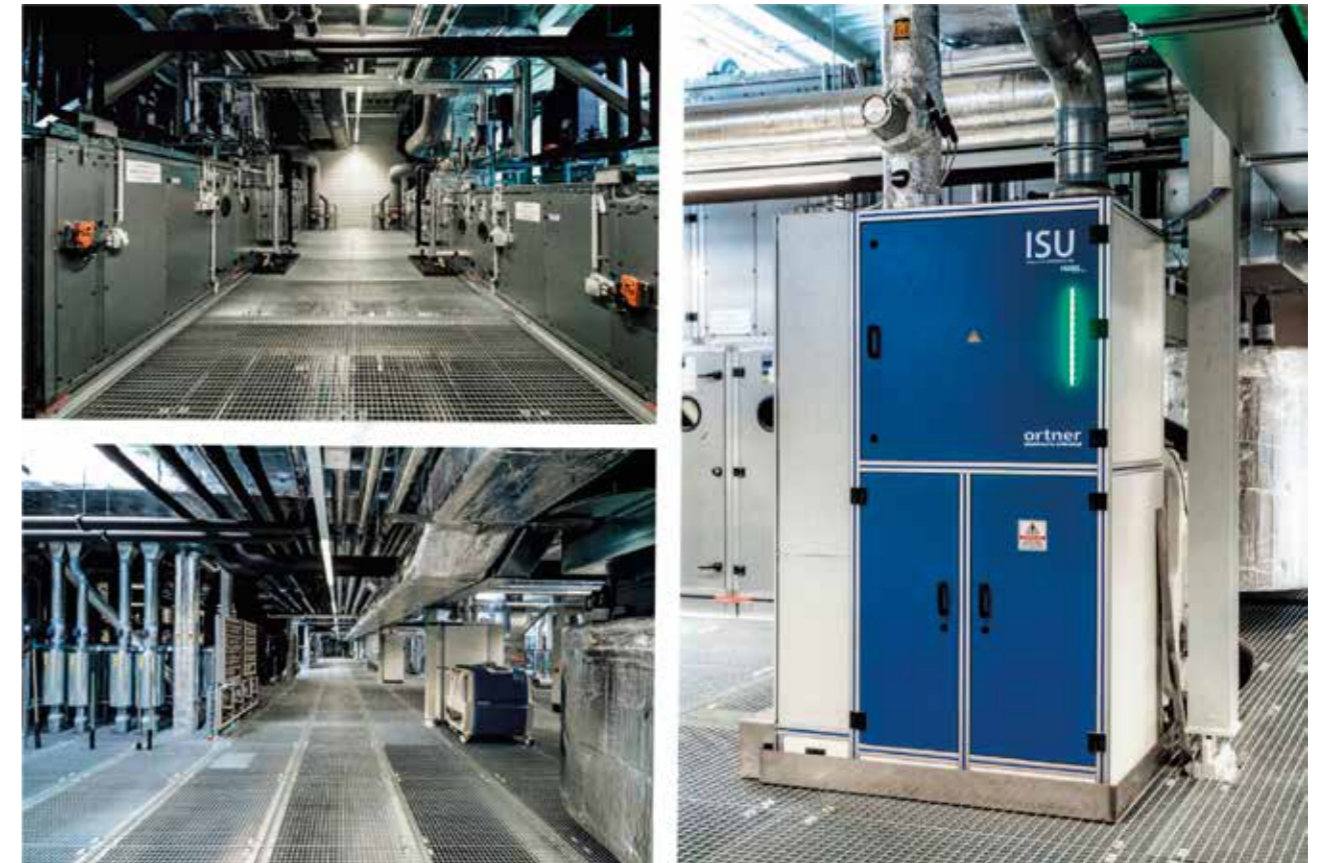
A fully automated decontamination system, which is positioned outside the clean rooms, centrally supplies the individual rooms.
