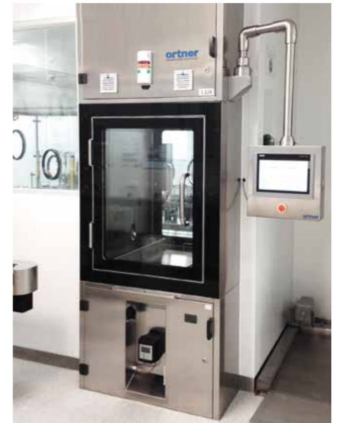
H 2 O 2 decontamination lock in the exit area
